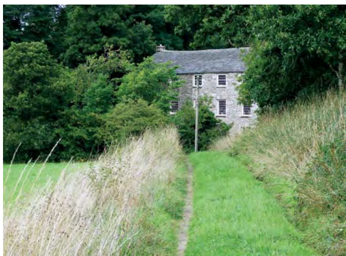
Track to Sprint Mill
